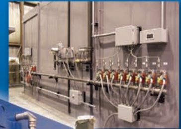
Vacuum Piping System w/Pressure Transducer & Thermocouple Jack Panel
